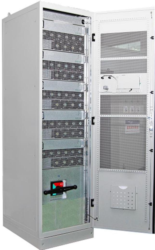
Figure 7-8 Cabinet's front ventilation holes
